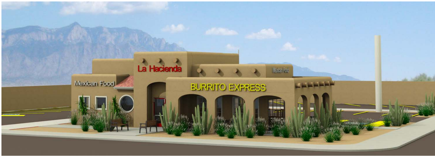
FRONT VIEW FROM CENTRAL (DINING/PATIO COLOR -I) DINING ROOM & PATIO COLOR I
